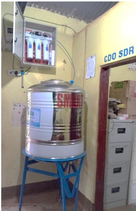
UV system in a Premium Cage installed with a sink and 400l smart tank at Mutufu CDC, Sironko
