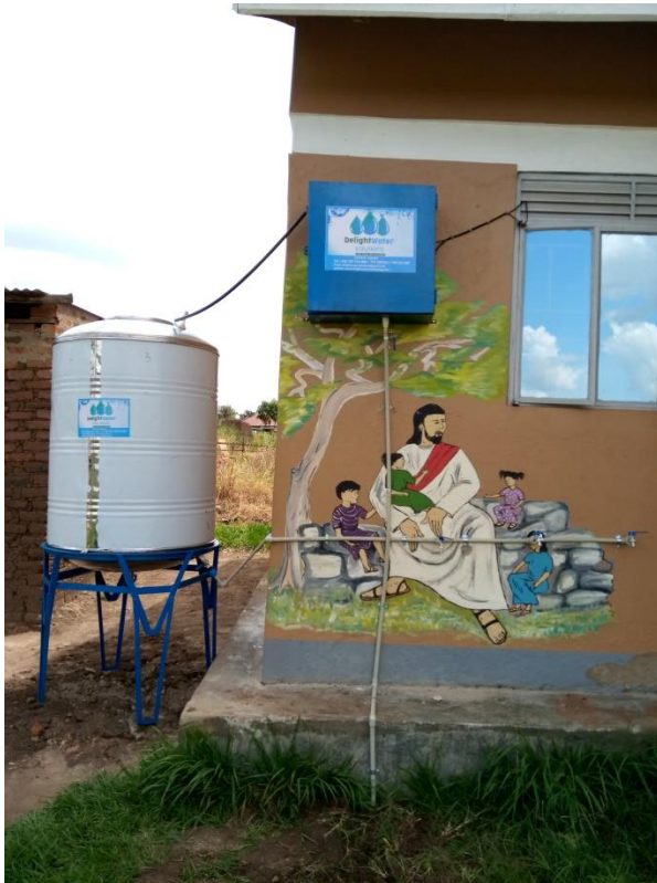
UV systems in a Standard cage (left) and Premium Cage(right) installed with 1000l and 450l smart tanks at Genrwot CDC Bweyale and Busolwe CDC Butaleja, respectively funded by Compassion International.
