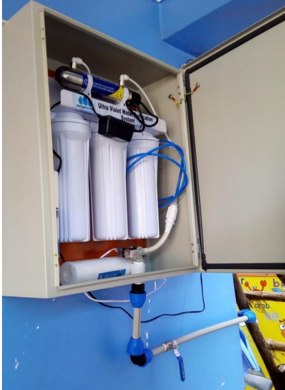
UV system in a Premium Cage installed with 1000l smart tank at Kampala Preparatory school, Kitebi
